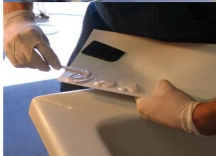
4b) Manufacturers prefer the acrylic filler. It is prepared by dispensing the desired amount of component "A" into a plastic graduated mixing cup. Add 30 drops of component "B" per each 1/2 ounce of "A". Mix thoroughly with the wooden stirrer, and use immediately, since it will harden within 15 minutes.
