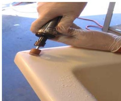
2) Remove all loose fragments from the edge by sanding with 100 grit dry sandpaper. Control the sanding to the immediate area of the crack to minimize the total area of the repair.
