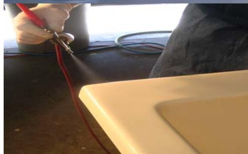
4) Allow the final coat to dry for 15 minutes before attempting to sand, buff, and polish. It can be wet sanded with 400 and/or 600 grit sandpaper to improve gloss and smoothness. Frequently, you can skip 400 and go directly to 600 grit.
