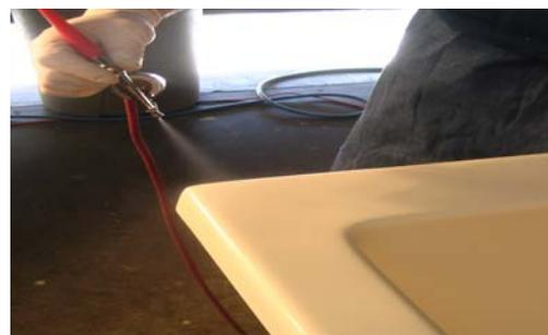
4) Now, use the K2000 thinner alone, as the finishing solvent to blend and wet out the “halo” effect in the feathered area. The airbrush should be held 8” to 12” from the surface during this operation. The heat gun can be used to accelerate drying. Allow the finished coatings to dry, and if properly applied in a clean environment, it should not require buffing and polishing.
